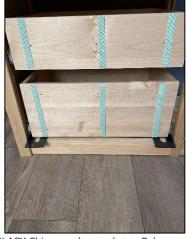
Starting with the first drawer, set the BLACK Shims as shown above. Balance them on the cross rail. These are 1/4"thick and will set the first gap.
