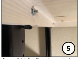
Secure all 4 bolts with washers and nuts. Secure the lock nuts on the ends of each bolt to prevent any nut from becoming loose over time.
